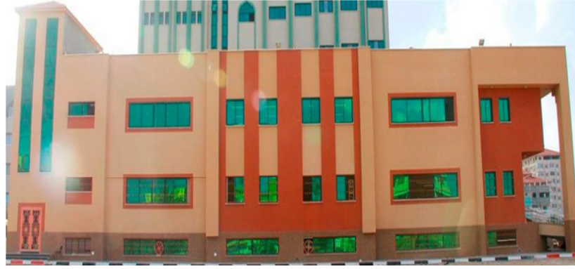
Figure 2.8: Irada building from west direction
