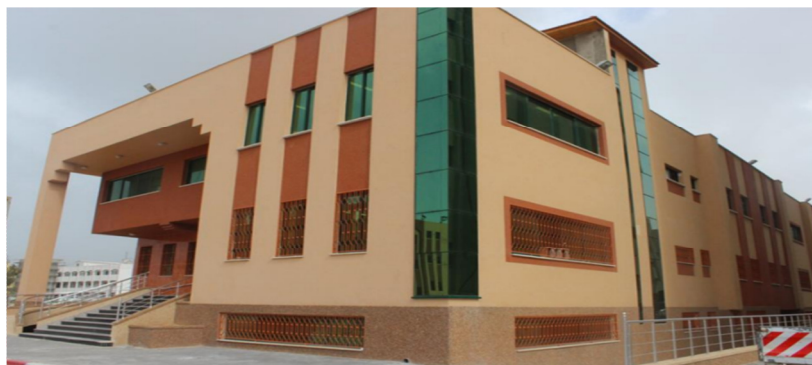
Figure 2.7: Irada building photo from south direction
